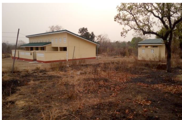
Figure 5.6: JICA Completed CHPS Compound at Kande, UWR
