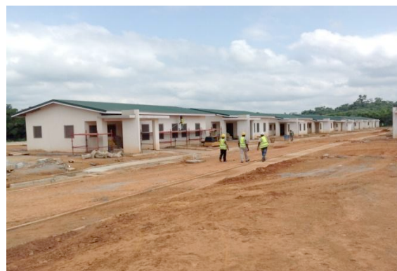
Figure 5.7: New District Hospital at Fomena, AR
