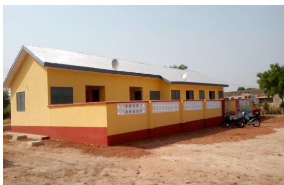
Figure 5.3: Newly completed CHPS Compound at Kunta, UWR
