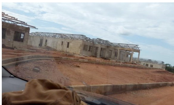
Figure 5.1: New Nsawkaw Hospital under Construction
