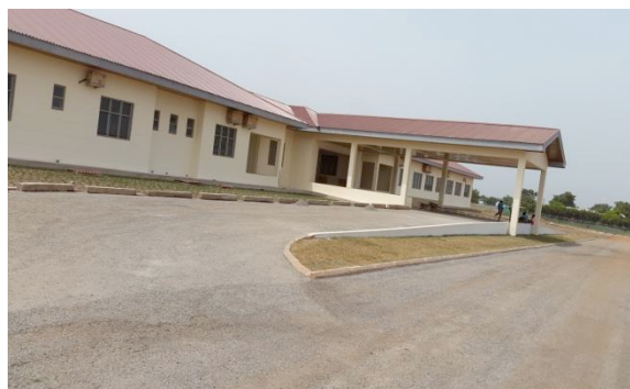
Figure 5.2: New Upper West Regional Hospital at Wa
