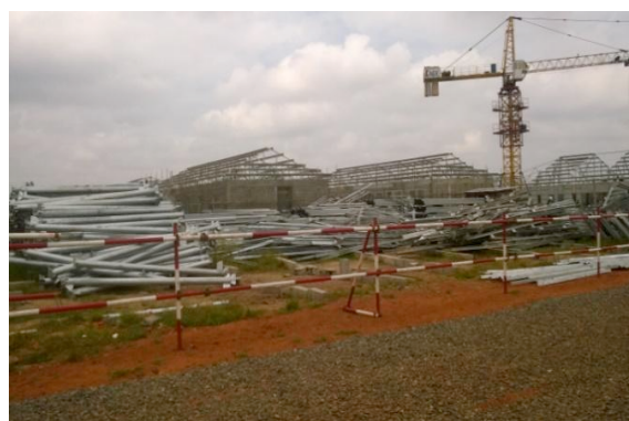
Figure 5.4: New Ga-East District Hospital at Kwabenya
